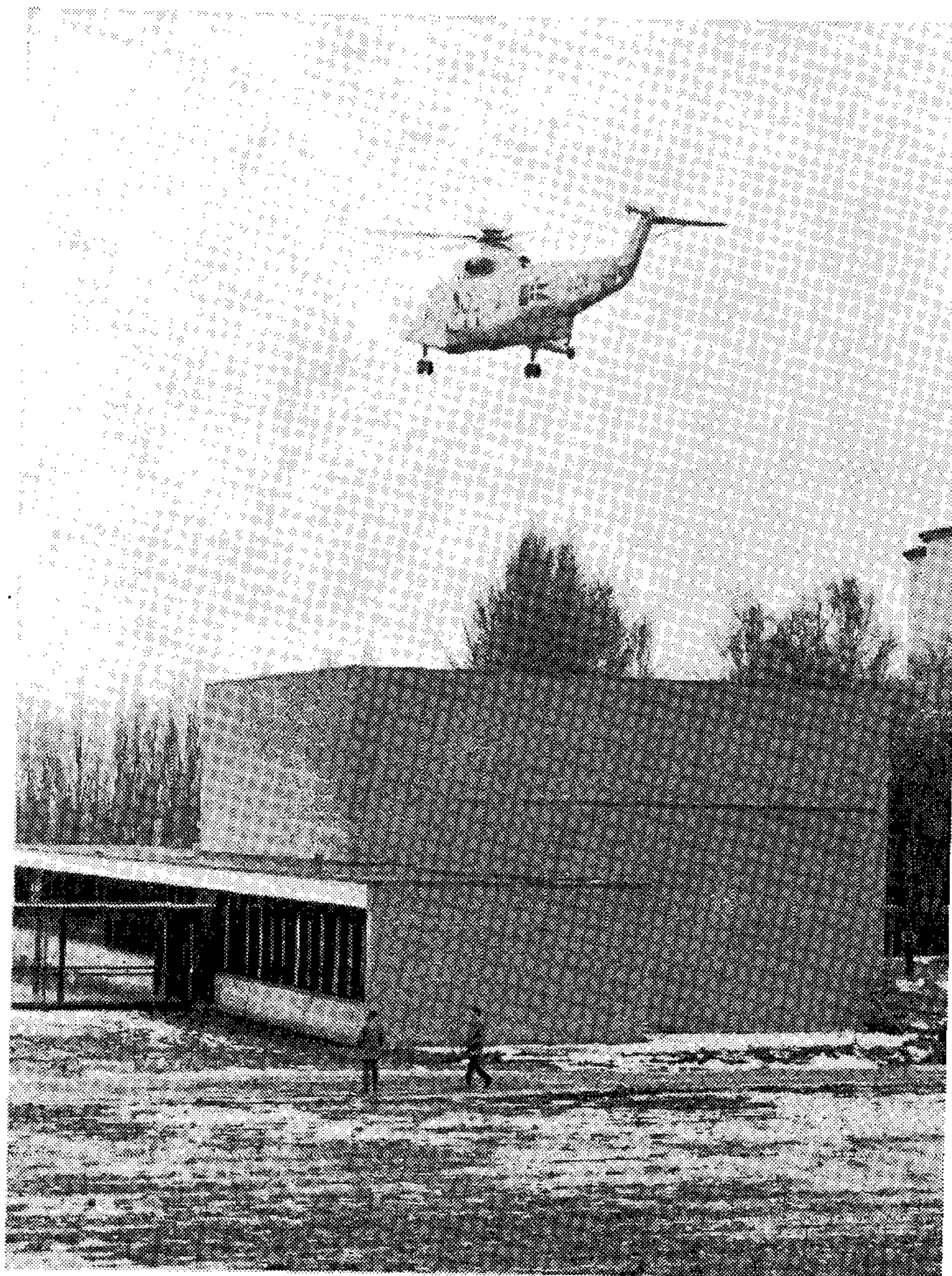
Fig. 24. "Sound source" used for measurement of the sound insulation properties of the double wall construction.
